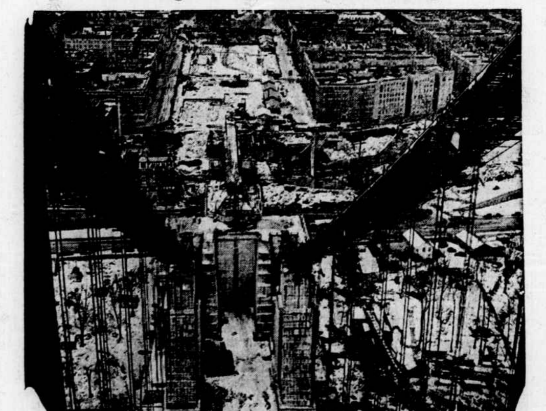
The east or New York anchorage of the majestic new Hudson river bridge, which connects the states of New Jersey and New York, as seen from the top of the bridge tower.
