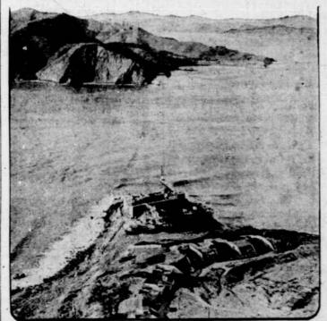
DRELIMINARY work for the construction of the giant Golden gate bridge at San Francisco is under way, as may be seen in this aerial view. The trestleway has been completed to allow work on the great calssons which will protect the foundation workmen who will fabricate the south pier in front of Fort Point. The white landmark on the far shore, Lime Point, is the location of the north nias.
