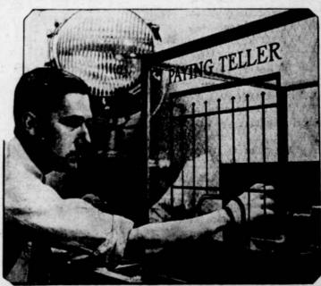
THE famous Westinghouse "electric eye," or photo-electric cell watchman, has been perfected to such a degree that Westinghouse has placed a \$20 bill in an exhibit at the World's fair in Chicago, free to anyone who can get it. The catch in the proposition is that as the hand is pushed through a min-lature paying teller's cage it interrupts a beam of light which in turn causes the photo-electric cell to raise a barrier instantly to protect the treasure it
