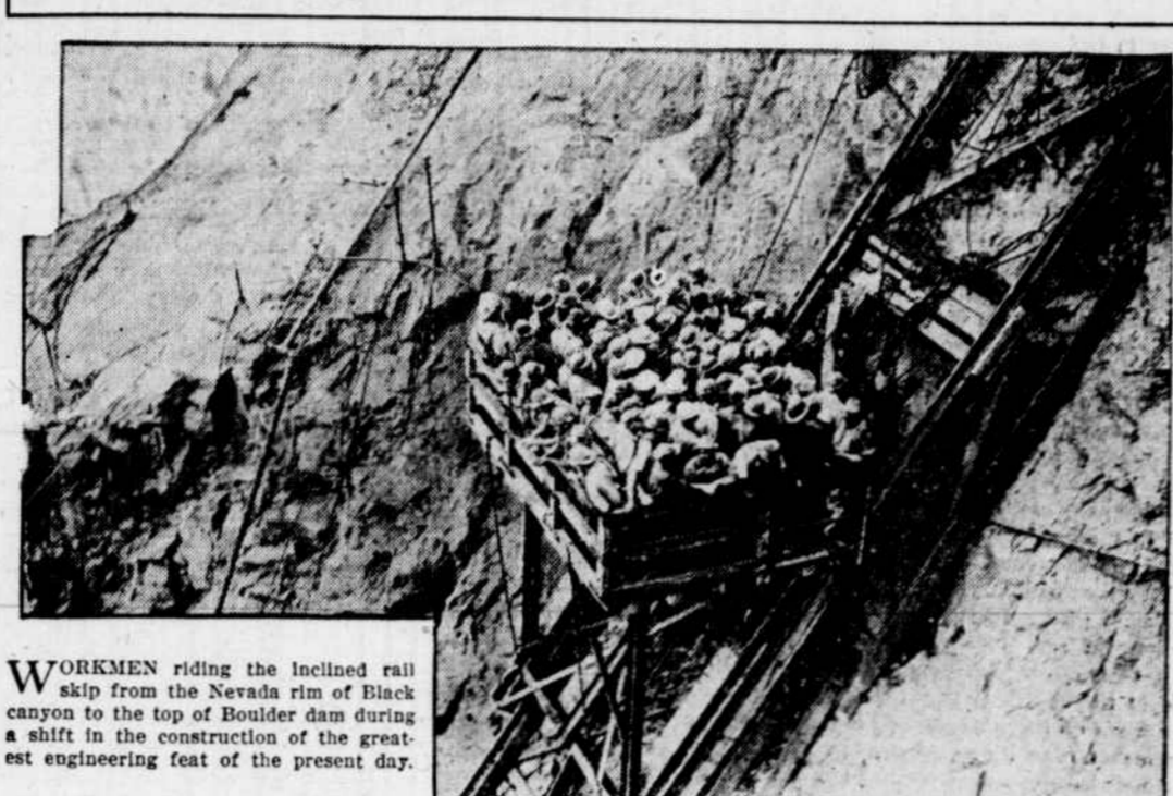
WORKMEN riding the inclined rail skip from the Nevada rim of Black canyon to the top of Boulder dam during a shift in the construction of the greatest engineering feat of the present day.
