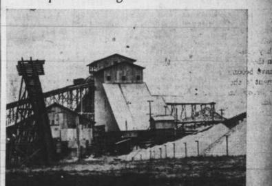
THE crushing sheds and piles of phosphate rock in central Florida. In this shed the hard rock phosphate is washed, dried and screened to various sizes. The phosphate industry is one of the state's largest.
