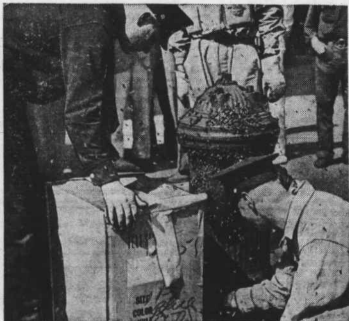
It was a good thing that a fire didn't break out in Detroit in the area of this fire hydrant which was taken over by a swarm of bees. Bee experts say the bees crossed the Detroit river from the Canadian side and decided that the fire plug would be a good spot to rest. Two Detroit policemen are shown trying to get the bees to move away from the hydrant.
