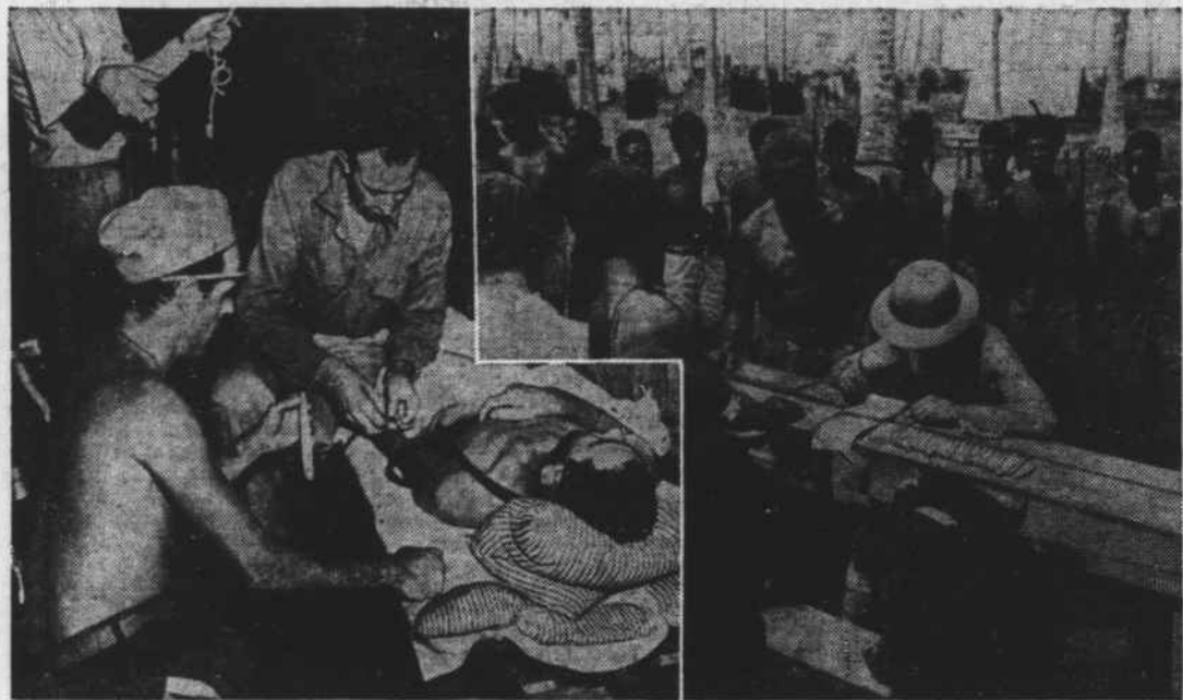
At the site of some of the bitterest fighting of the war, a senior medical officer of the United States naval construction battalion is shown, at left, giving a blood transfusion to a Seabee in a foxhole on Guadalcanal island in the Solomons. At right, several husky natives line up to receive their pay as stevedores. The Seabees—men of the naval construction battalion—are making a base of this island which was wrested from the Japanese after a long battle in which both sides suffered heavy losses in planes, ships, and men.
