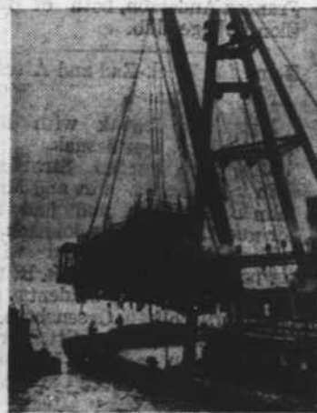
Salvage work is in progress elsewhere also. A bridgehouse from a sunken ship off Staten Island is hoisted to a barge.
