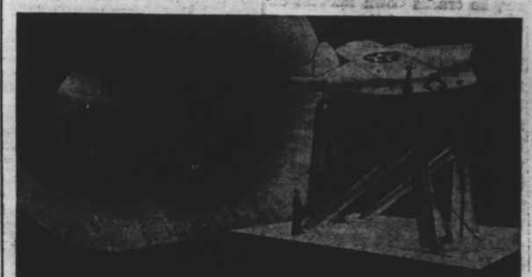
A FIGHTER PLANE, the Brewster XF2A-1, is shown mounted on struts in the full scale wind tunnel, ready for testing. The struts are connected to instruments in the room below the platform, which record the various stresses which the plane undergoes in this largest wind tunnel in the world. (All pictures are official photographs released by the National Advisory Committee for Aeronautics.)
