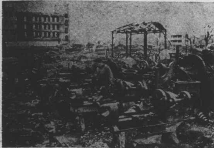
Home as well as factory industrial facilities felt the lash of U. S. air raids, with only the machinery standing in the ashes of this burned-out residential shop in Tokyo.
