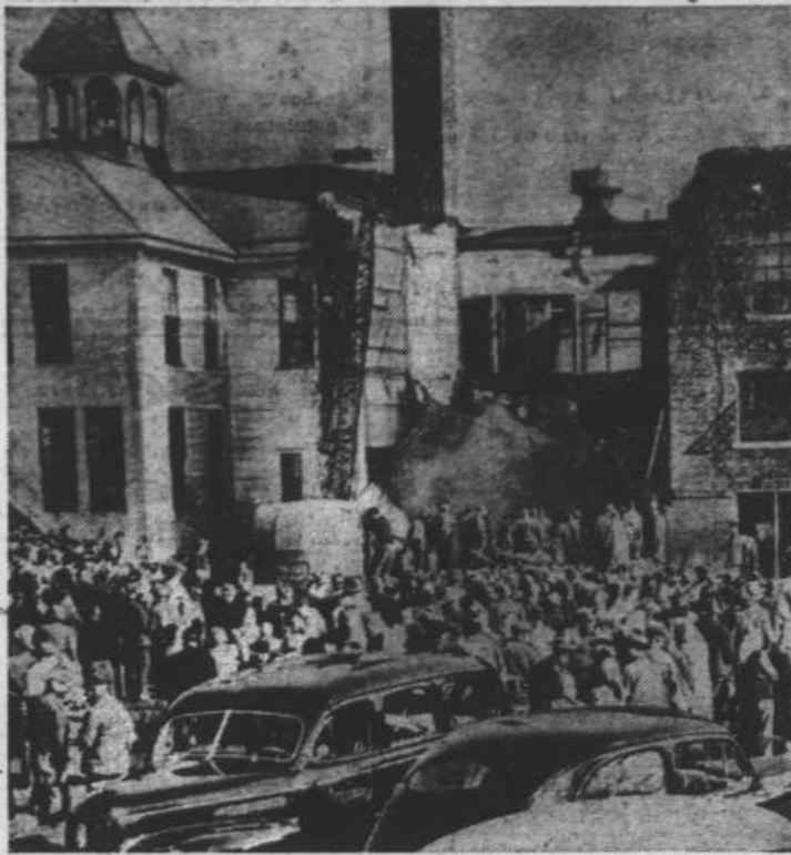
BLAST WRECKS SCHOOL . . . Crowds of anxious parents and volunteer rescue workers gathered quickly at the Baroda consolidated school at Baroda, Mich., following a boiler explosion in the basement of the school which killed one child and injured at least 16 others. When reports were first received at Chicago rescue planes with medical supplies were rushed to the scene.
