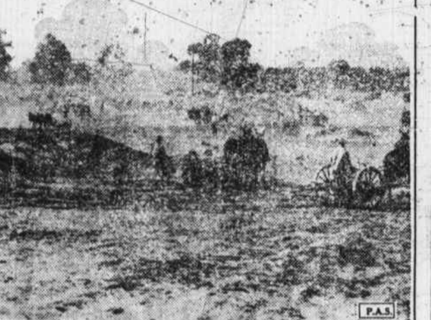
OCALA, Fla. . . . Hundreds of mule-drawn scrapers are biting into Florida soil, digging the path which will be a sea-going ship canal across the state, joining the Gulf of Mexico with the Atlantic Ocean and thus taking coastwise ships out of the hurricane zone around the keys.
