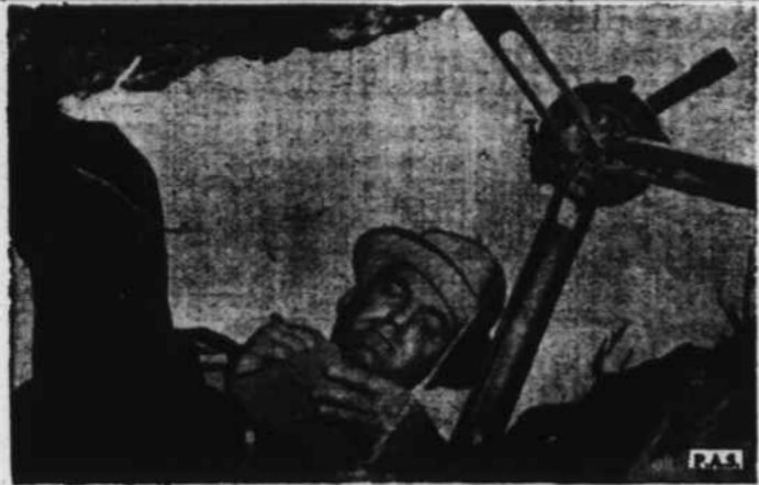
Here's a worm's-eye view of an avalanche in the making. Lowering himself into a huge fissure at the top of the "moving mountain" in Los Angeles' Elysian Park, a daring cameraman shows how the ever-widening crack is being checked hourly to determine course and extent of the next in a series of huge earth-slides that have already sent millions of tons of rocks, earth and trees tumbling 850 feet into Riverside Drive, Dayton Avenue, below, and even into the dry bed of the Los Angeles river, 1,000 feet away.
