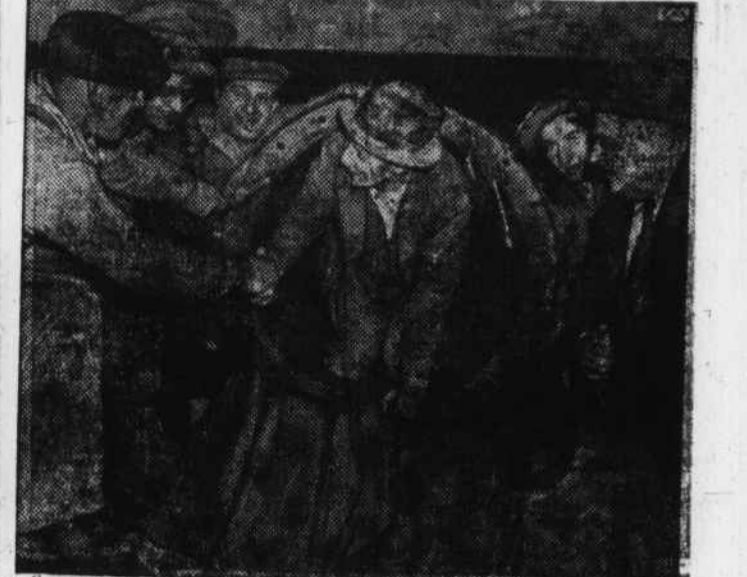
Hundreds of feet below the waters of the Hudson, the north tube of the Lincoln Vehicular Tunnel is 'holed through' to connect New York and New Jersey. The tunnel is designed with two tubes, each one-way. The south tube is already in use. The north one will be completed next year. As a climax to the two-year digging job, sand-hog crews from each shore meet near center of the river bed.
