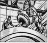
1. The new million volt X ray 2. Defects in the steel show up on built by General Electric saves X-ray film. Therefore faulty mateprecious hours in finding flaws. It is so powerful that its rays can pierce hours of machining have been spent thick steel castings.
