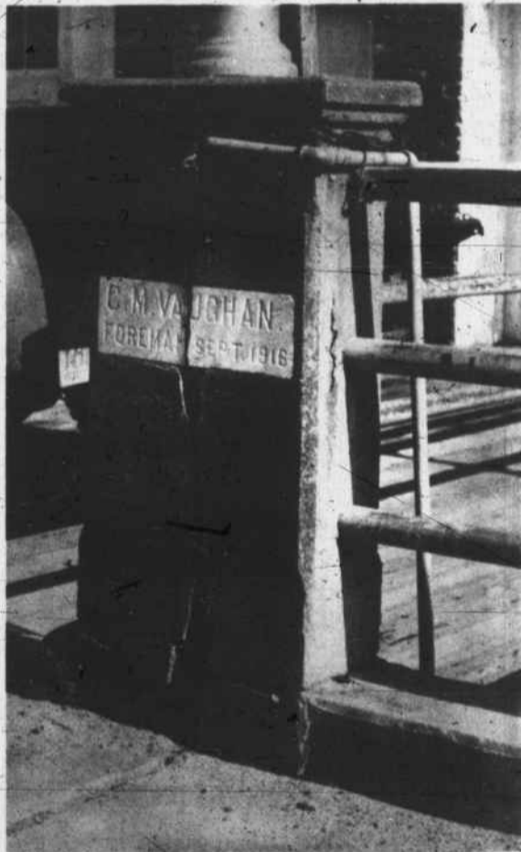
1916 Vintage Even the corner stone of the 1916 vintage Main Street Tar River Bridge here gives mute testimony as to the present state repairs the bridge is currently in. - Times Photo.
