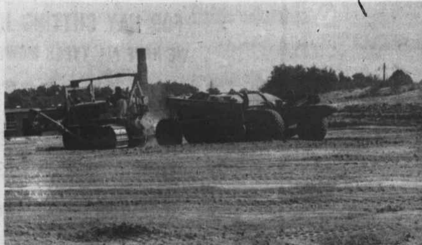
Work On School Playground
