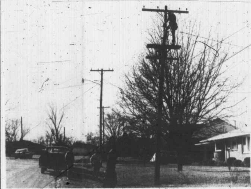
New Lights Installed
