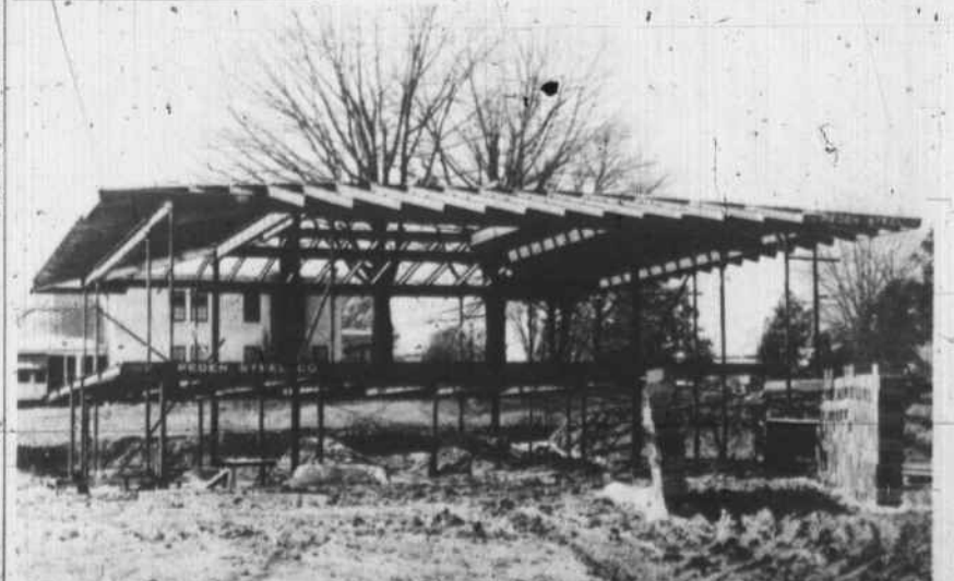
New Bank Building Construction
