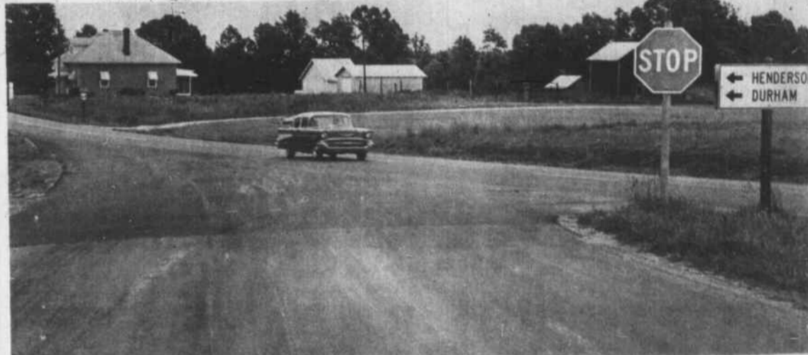
This is N. C. 98 at the intersection of U. S. 64 east of Bunn. The point shown is .55 miles from the Franklin line inside Nash County. Still another case of improved roads near the Franklin County line.
