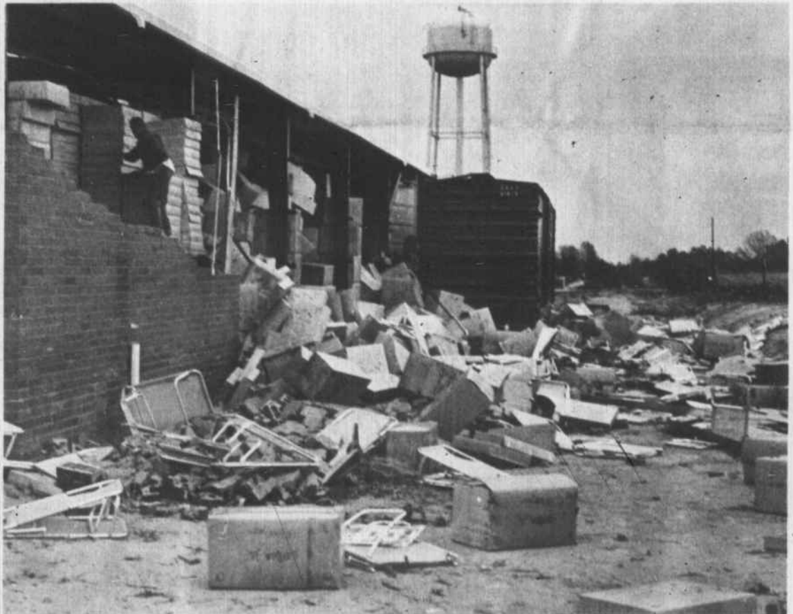
Where Tornado Struck Part of the damage to the Gay Products plant can be seen above, following the 3:10 p.m. tornado which tore out the south wall of the one-story building. Aluminum chairs were strewn over a wide area by the storm and power was disrupted at the plant on N. C. 56 west of Louisburg. There were no injuries reported, but damage was heavy.
