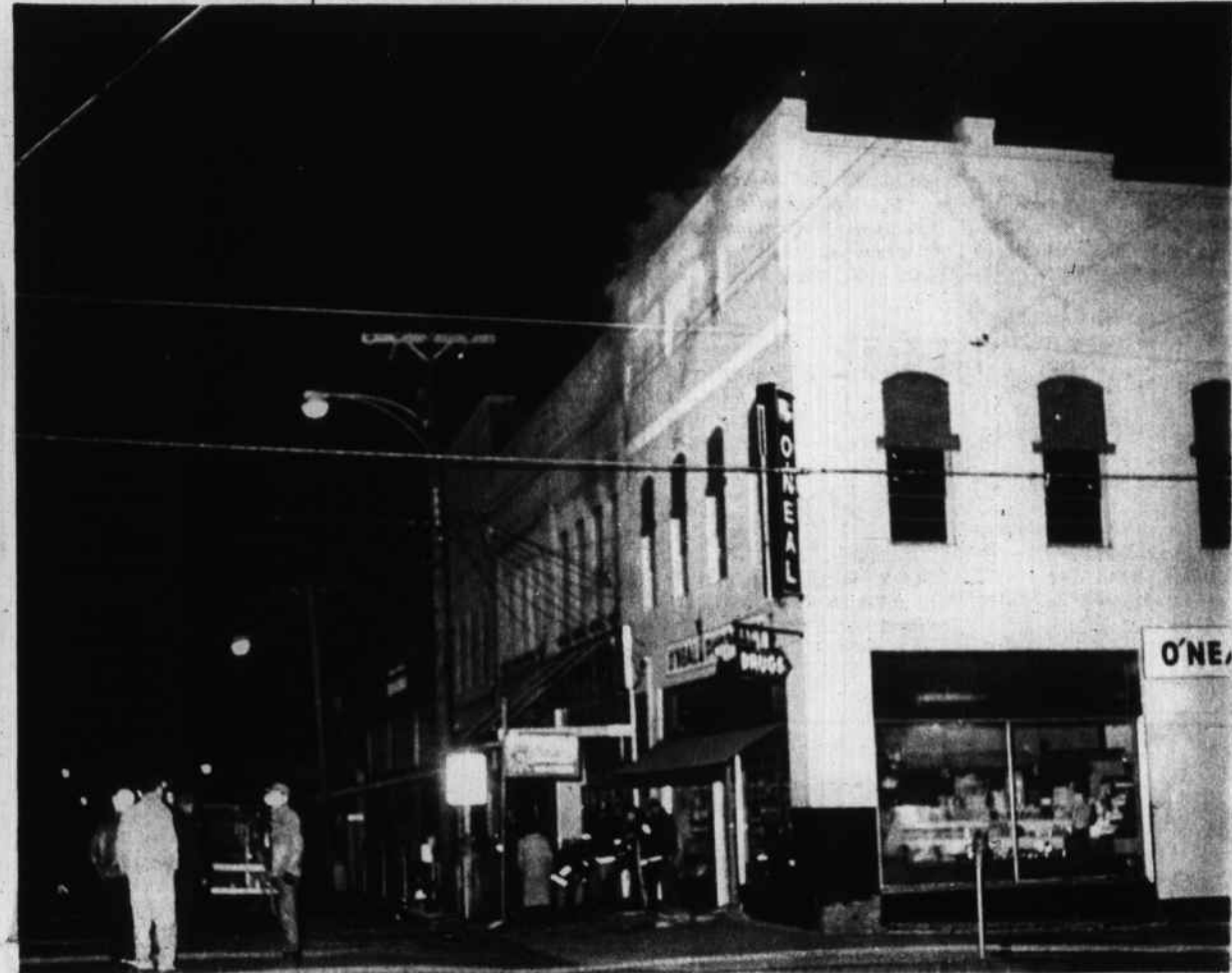
SMOKE POURS FROM ROOF AND WALLS OF BODDIE BUILDING AT HEIGHT OF FIRE TREAT EARLY WEDNESDAY MORNING.
