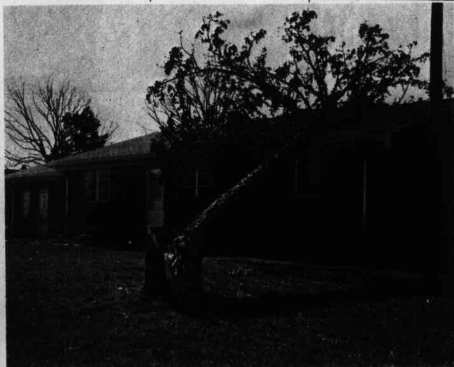
Home Damaged At Justice
