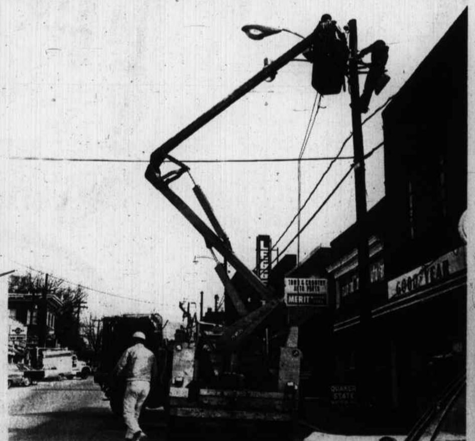
Franklinton Gets New Street Lights
