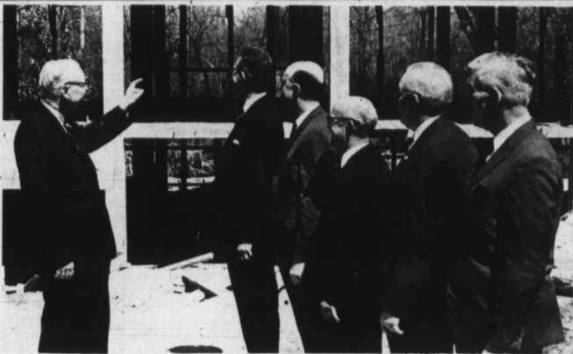
Board Of Visitors View Construction
