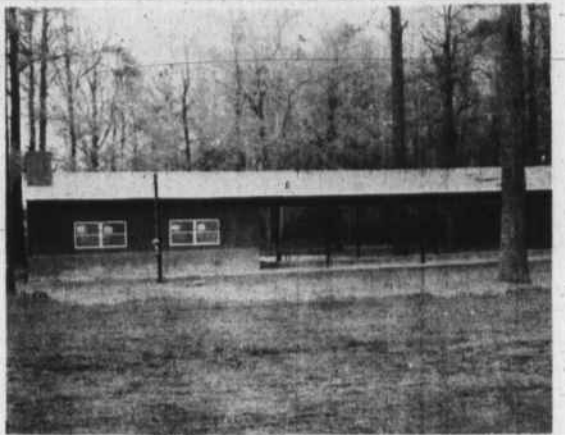
Shown above is the picnic shelter and meeting rooms built by the Pilot Baptist Church Recreation department. The 90' x 24' foot structure cost around $5,000. The organization is staging a barbecue supper Saturday night at Pilot to raise funds to build two asphalt covered tennis and basketball courts. Future plans call for lighting a little league baseball and softball field.
