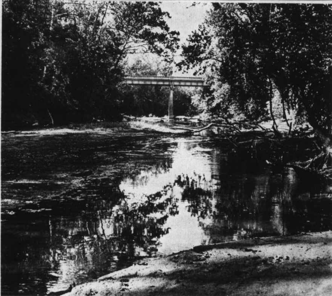
This Is The Tar River Below Bickett Bridge
