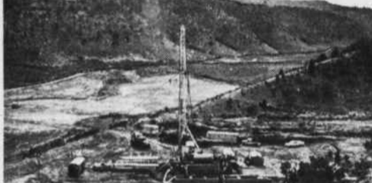
COLORADO may be "oil country" as Oil Shale Corporation takes cores to determine thickness, quality, depth of oil-bearing shale beds. Hilly tract is government-owned.
