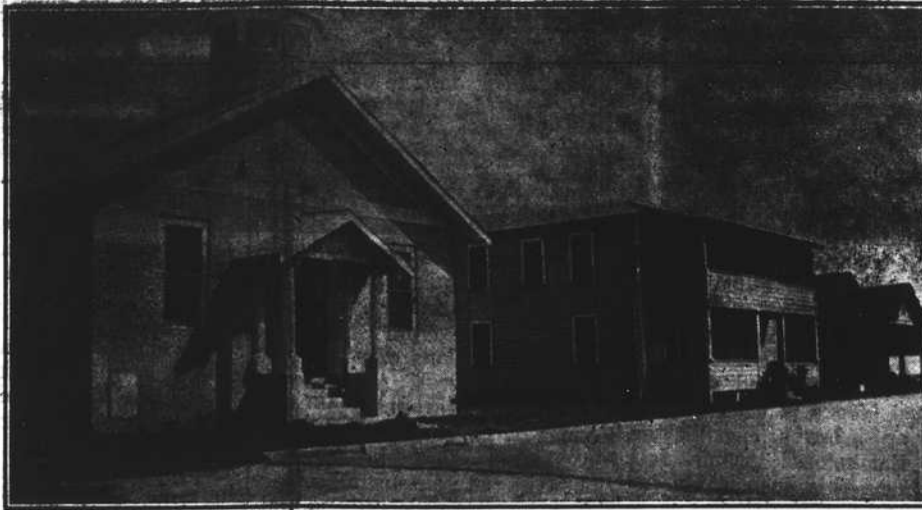
GOOD WILL CHURCH AND MANSE AT FORT PIERCE
