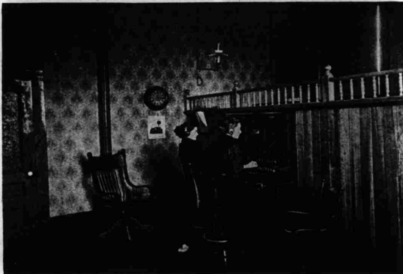
GREENSBORO TELEPHONE EXCHANGE.
