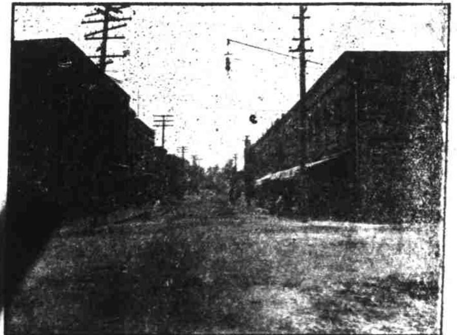
SOUTH MAIN STREET FROM THE INTERSECTION OF FOURTH.
