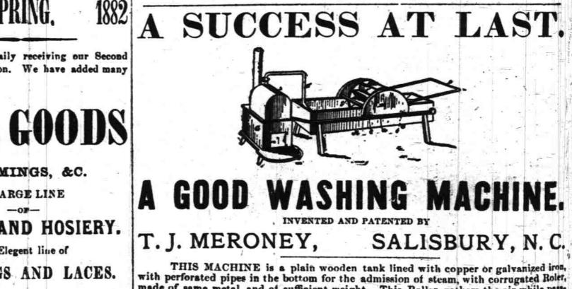
made of same metal, and of sufficient weight. This Roller gathers the air while passing back and forth over the clothes, forcing air and water through the fabric. At same time the steam is thrown up through the perforated pipes underneath from the bottom of the tank. There are wooden strips between the pipes so as to protect them and form a smooth bottom in the tank.
