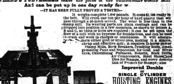
We construct Mills with Stamps weighing from 350 to 900 lbs. for gold and silver ores. Wet or Dr. Crushing Mortars. Send for Circular. Wal 8:00 ms 9 and 84 Like rty 511661, New York.
