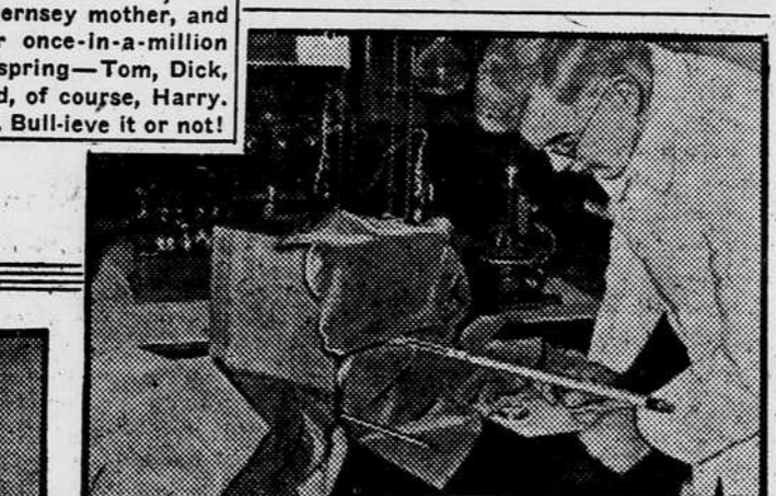
FABRIC THAT BREATHES—Exhaustive tests all new auto features go through are indicated in this picture of a Pease laboratory scientist examining new "breathing back" mohair velvet upholstery introduced on 1936 Fisher bodies. The fabric loses heat quicker than former simiac materials.
