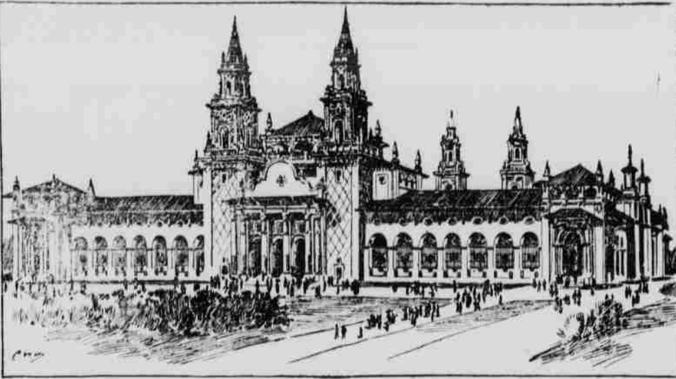
Copyright, 1900, by the Pan-American Exposition Co. This fine structure is 500 by 450 feet, with a central court 100 by 175 feet. Its type of architecture is the Spanish Renaissance, modified to suit the conditions of the Exposition. The roofs are laid with red tile and the cemented walls are brilliant with color. The colors are to be reds and yellows in light tints. The facades will present an arched effect, with broad, overhanging eaves, in imitation of the old mission buildings in California and Mexico. The central court will be a veritable tropical garden, with a long, narrow pool, containing interesting specimens of aquatic life, and will have seats, where the weary visitor may rest a moment. The Exposition is to be held in Buffalo in 1901 from May 1 to Nov. 1.
