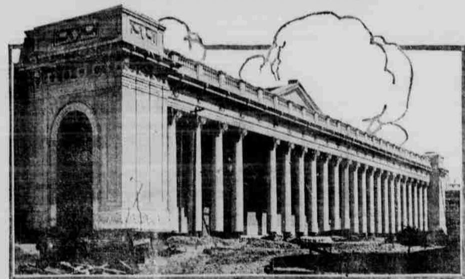
Copyright, 1914, by Panama Pacific International Exposition Company. Colonnade, entrance of the Court of the Four Seasons upon the esplanade on San Francisco harbor and extending the west facade of the Palace of Agriculture. One of the columns of the colonnade has been temporarily removed to permit freight trains to enter the palace. Panama-Pacific International Exposition, San Francisco 1915.
