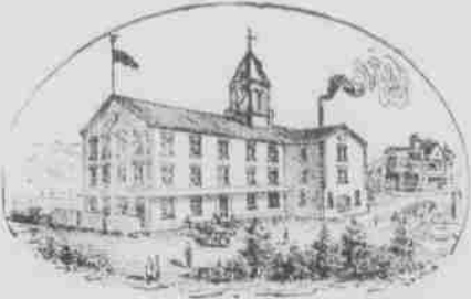
Paper Product Company's Plant Destroyed by Fire Sunday morning Building was Owned by Garrett & Company, of Norfolk.
