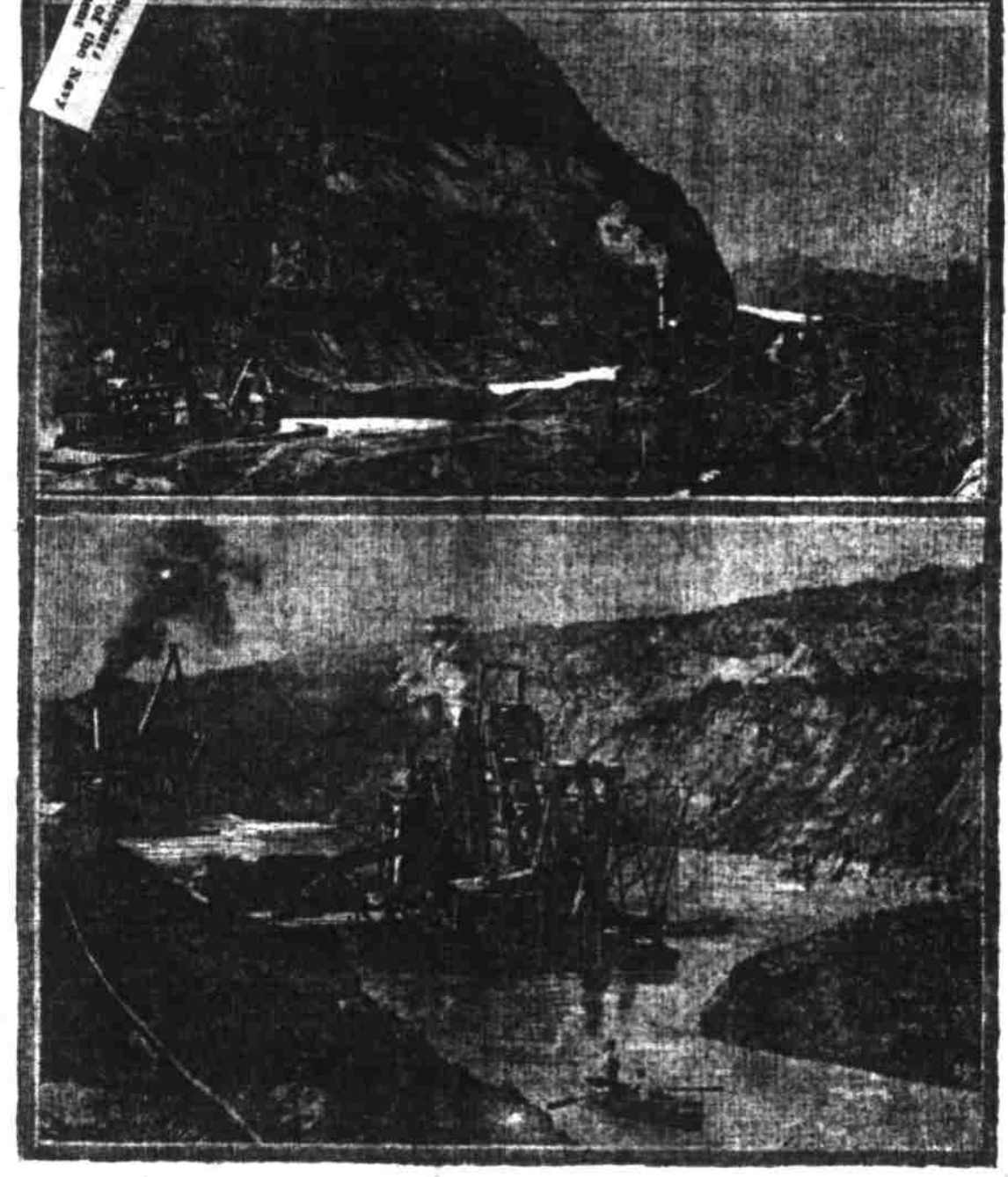
Narrow channel which must be dug out every day to permit row boat passage. These photographs show the stupendous work ahead before Panama Canal can again be opened to navigation. Thousands of tons of earth and loose rock slid down from Gold Hill at the left as shown in the upper photo and completely blocked the canal, which was 200 feet wide at this point. The lower picture shows the dredgers at work keeping clear the narrow passage which permits a row boat to get through. This fills every day from the mud rising in the bottom, due to the pressure of the hills on the side of the cut.
