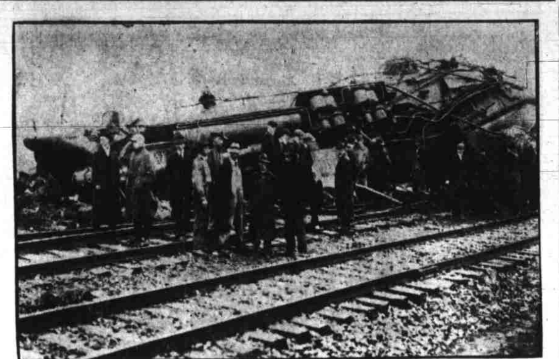
Lying diagonally across the main line of the Seaboard, the big boiler rested after being hurled a distance of more than a hundred feet by the force of the explosion. It did not burst except under the bottom, appearing to have been lifted bodily from its moorings on the trucks. This picture was taken immediately after the wreck.
