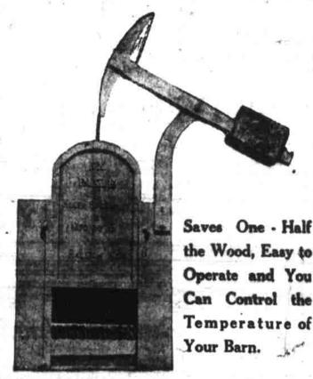
Equipment consists of one complete front; six grates 6"x30" and one grate rest. This makes the fire box 18'x60". Furnace can be made longer by putting in extra set of grates. The door is controlled by the weight, making it self-balancing. The "Dixie" is the most complete operating furnace on the market.
