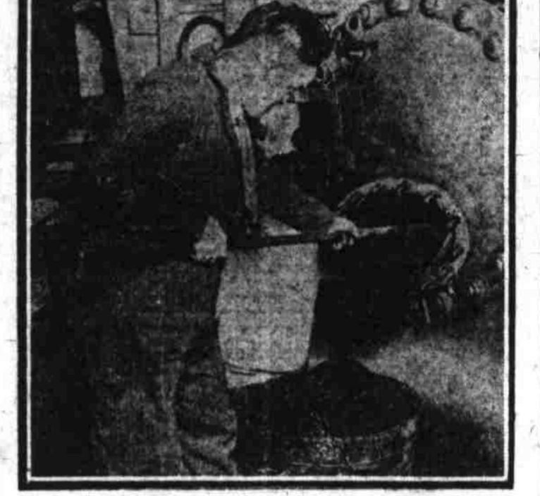
Government experts of the forest products laboratory of the Department of Agriculture in Madison, Wis., have developed a new stock food from sawdust. The photo shows the cylinder in which the food is made. Fifteen minutes cooking in this cylinder with diluted acid under steam pressure converts a part of the wood into sugar and renders the remaining digestible.
