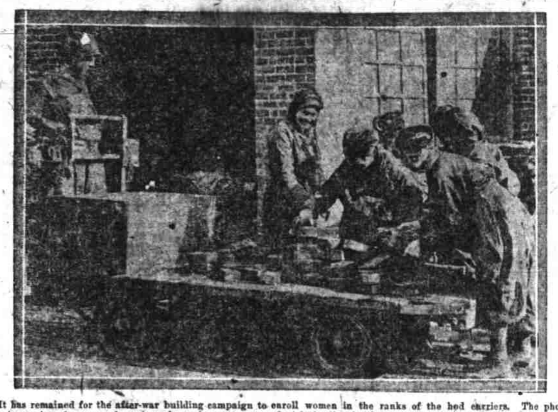
It has remained for the after-war building campaign to enroll women in the ranks of the hod carriers. The photo, made in an American manufacturing plant, shows women and girls loading brick on an electric conveyor.
