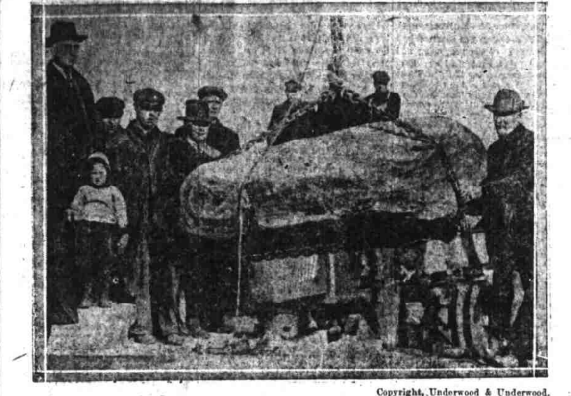
Copyright, Underwood & Underwood. Photograph shows the famous Plymouth Rock being moved to a new foundation just before the celebration of the tercentenary of the landing of the Pilgrims at Plymouth, Mass., a few days ago. The little boy beside the rock is William S. Brewster, descendant in the ninth generation of Elder Brewster, of Pilgrim fame.
