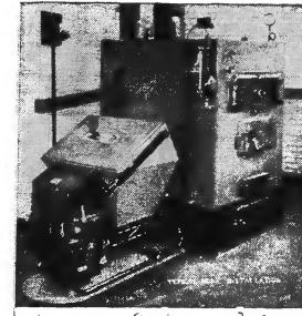
STOKOL is the world's greatest automatic stoker. It will reduce your coal bill from 20 to 50 per cent. It is constructed to be used with any standard type furnace, and is unusually easy to operate. It is not too late to have a STOKOL installed in your home. We will be pleased to make specifications and quote
