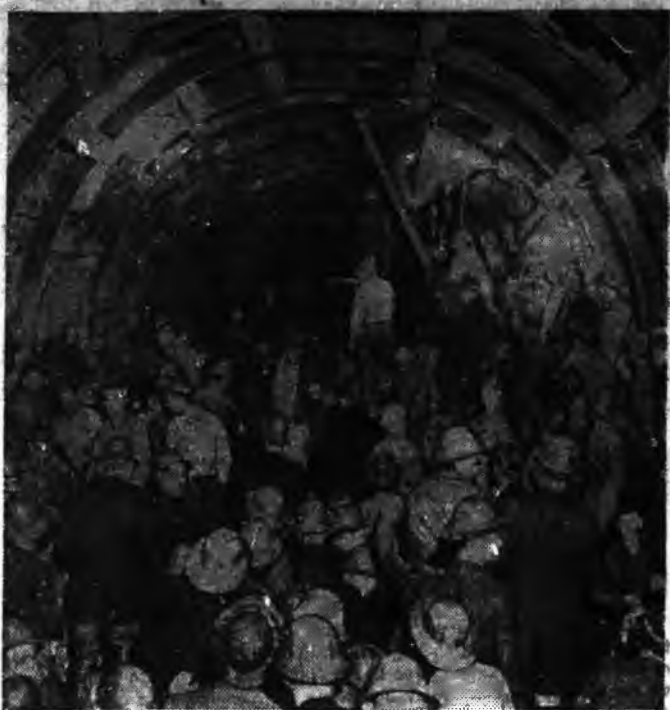
Completing a five-year job, hard-rock men boled through in the San Jacinto tunnel recently. Within a few months 1,000,000,000 gallons of the Colorado river will rush through this 13-mile bore daily in its haste to quench the thirst of Los Angeles and 12 other southern cities. It was one of the biggest tunneling jobs ever attempted.
