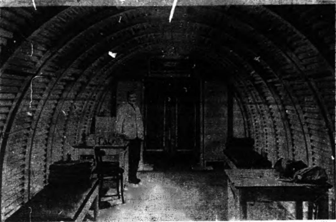
When—and if—the next war breaks out, London residents will be prepared. A specimen steel-lined shelter, built for use as a first-aid and dressing station underground in case of an air raid, can now be bought by private individuals or communities. The bomb shelter is a part of the national defense plans.
