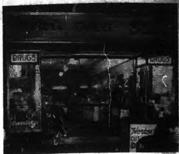
A front view of Horton's Drug Store, which celebrated its 40th anniversary Friday with formal opening as a highly modernized store. Note the attractive front and the brilliantly lighted interior.
