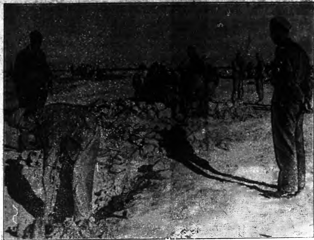
GERMAN PRISONERS, taken in the recent Allied reconquest of Eastern Libya, are put to work behind the Allied lines to build new roads and repair the towns and fortifications which were destroyed in the fighting. The men who guard them are Poles—members of the Polish Middle Eastern force which took such an important part in the drive to Benghazi. These men have families and friends back in Poland whose lot, under German rule, has been one of starvation, disease and forced labor—yet military discipline forbids the Polish soldiers from showing the pleasure they must be feeling at making the Germans work for them for a change.
