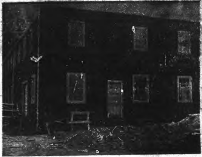
Model Upholstery company, a comparatively new local industry, has moved into the spacious factory building shown above, which is located just north of this city on highway 18. Arvil Phifer is head of the firm, which makes upholstered furniture. (Photo by Dwight Nichols)
