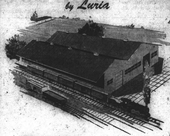
ERMANENT, all steel structures adaptable to any industrial, warehouse or commercial use erected in 1/3 to 1/2 time needed for ordinary buildings.
